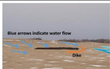
A dike can be constructed between the manure pile and a stream to minimize impacts to surface water. Dikes should be constructed out of soil, not organic materials.
