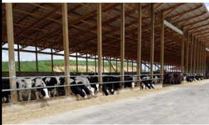
Monoslope buildings are popular in the Midwest for housing Holstein steers in cold climates and facilitating manure nutrient management. (Ramthun Farms, West Bend, WI)
